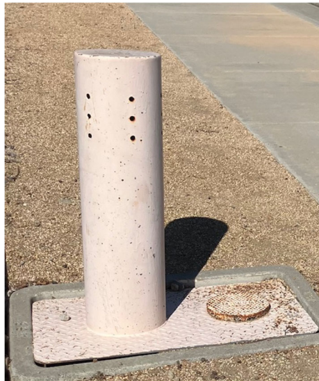
Figure 3. Typical Air Release/Air Vacuum Valve at Grade
